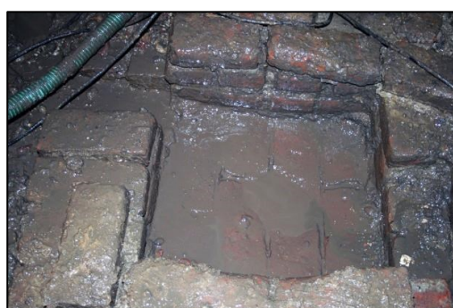
Plate 10: Brick Built Structure (Context 109)
