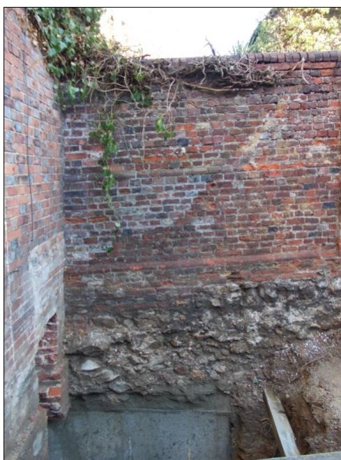
Plate 4: Garden wall with brick rubble footing
