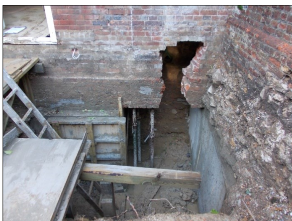
Plate 1: External excavations for the stairwell Plate 2: Internal excavations for the stairwell
