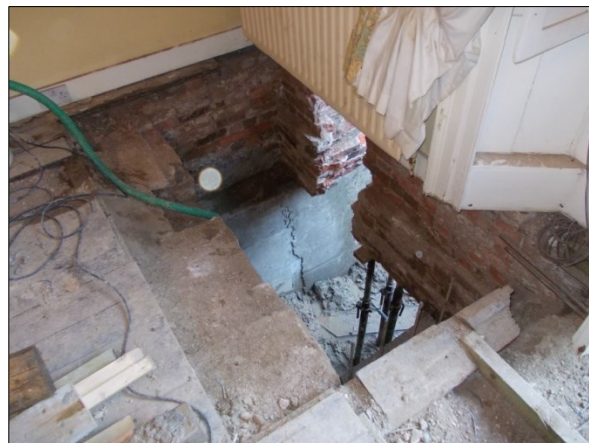
Plate 1: External excavations for the stairwell Plate 2: Internal excavations for the stairwell
