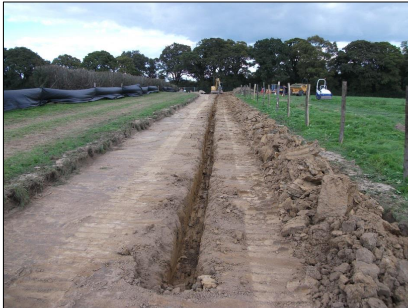
Plate 1: Roadway topsoil strip and service trench
