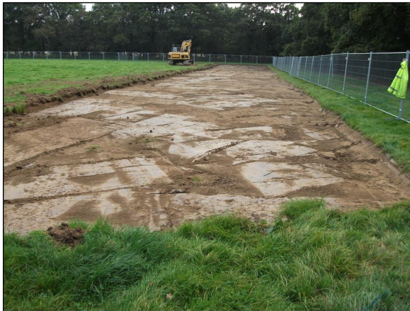
Plate 2: Machine stripping on the main part of the site
