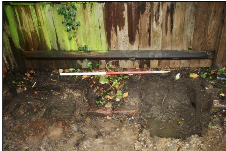
Plate 2: Trenches A and B
