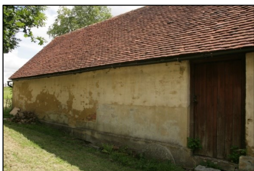
Plate 14: Western Elevation of Stable Block
