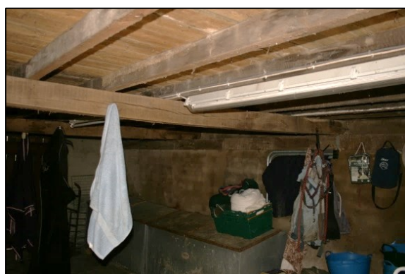
Plate 10: Ceiling of Ground Floor of Store/Barn
