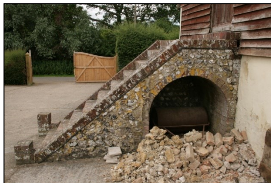
Plate 3: Arched Feature in Northern Wall of Staircase
