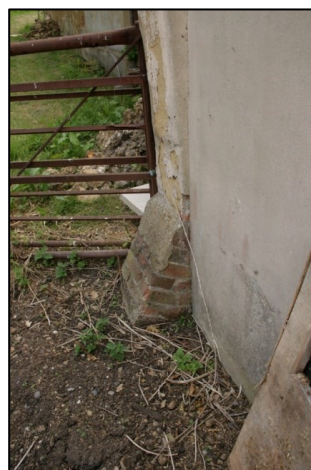
Plate 9: Buttress on End of North Wall
