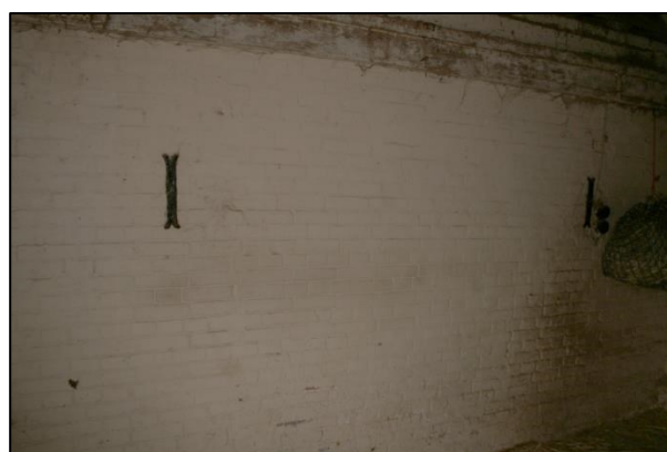
Plate 7: Wall Tie Plates in Southern Interior Wall of Stable Block
