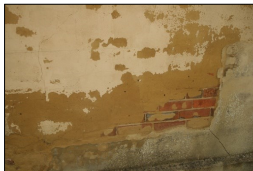
Plate 15: Exposed Brickwork West Wall
