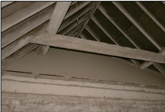
Plate 16: Roof of Store/Barn Visible in Southernmost Stall
