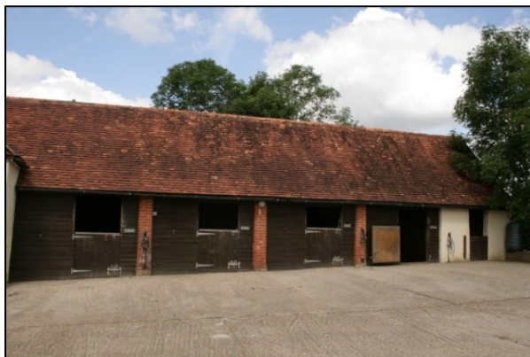
Plate 12: The Eastern Elevation of the Stable Block
