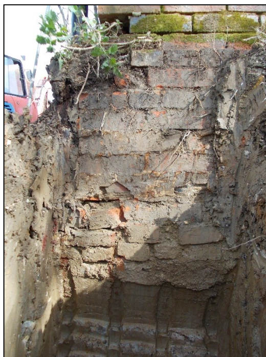
Plate 26: Brick foundation on NW corner of the Stable block
