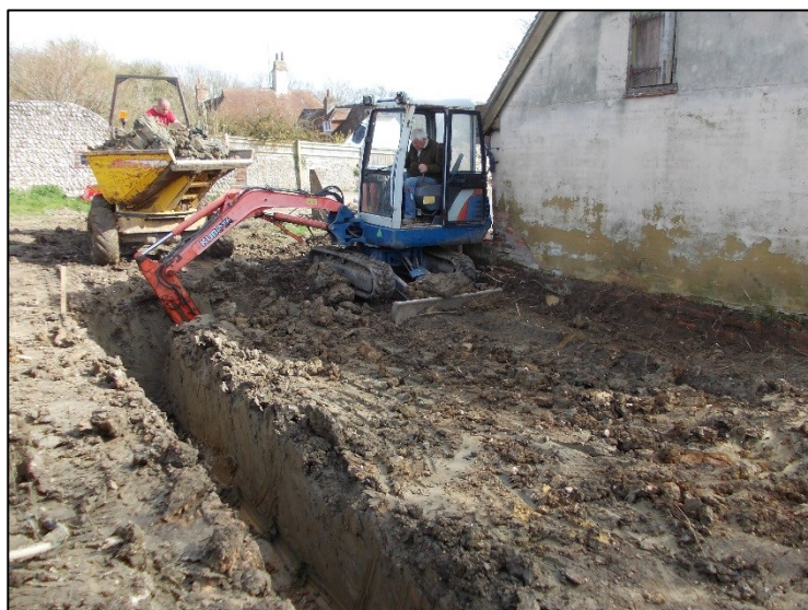
Plate 24: Excavation of the foundation trenches
