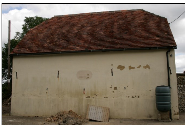
Plate 4: Southern Elevation of Store/Barn
