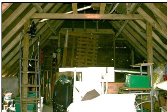
Plate 11: Construction of the Roof of the Store/Barn
