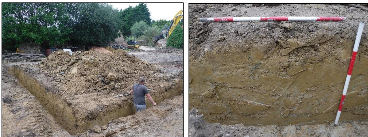
Plate 3: Excavating foundation trenches and section of foundation trench
