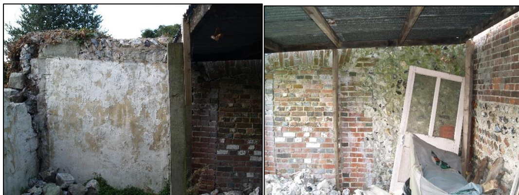
Plate 10 – Western internal elevation of G2 showing the plastered and painted wall to the south (left) and the blocked doorway and flint construction to the north (right).
