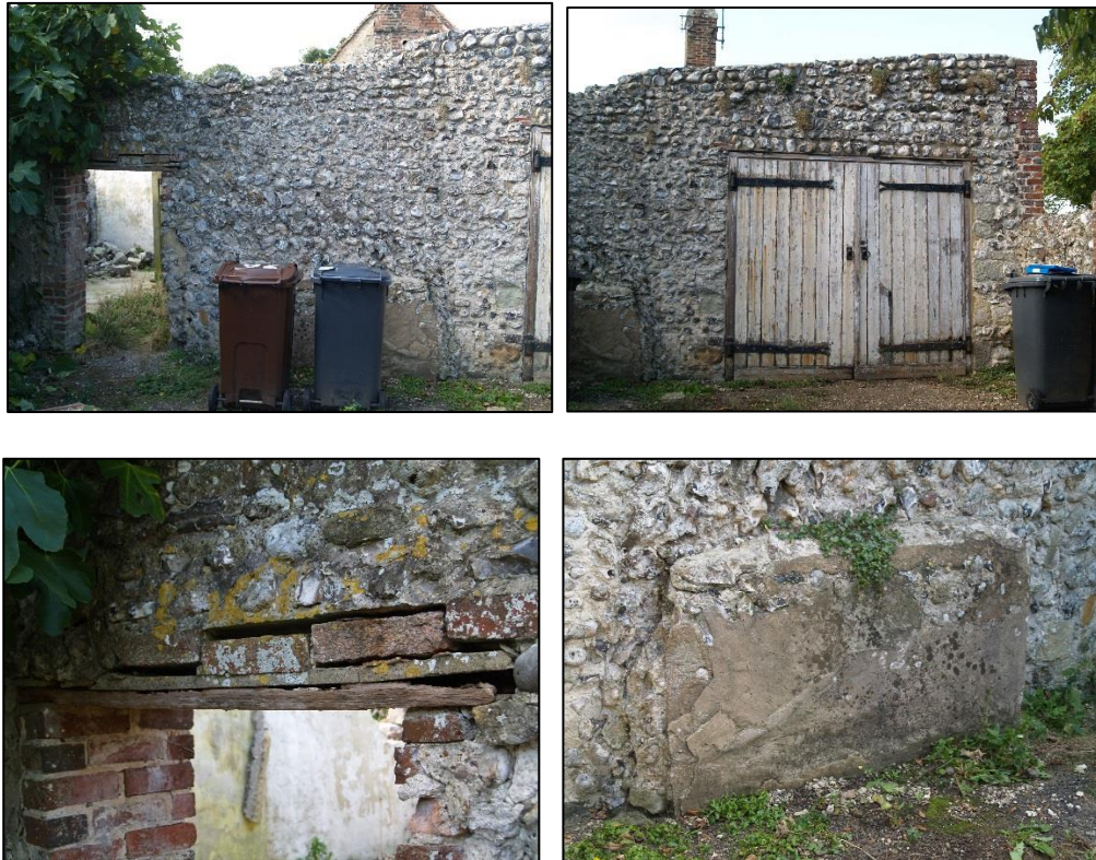
Plate 3 – The Eastern Elevation showing the doorway into G2 and wall to the south (top left) and double garage doors adjacent to the boundary wall, to the north (top right); note the change in mortar colour between G1 & G2. Detail of the lintel over the doorway into G2 (bottom left) and the small plinth (bottom left)
