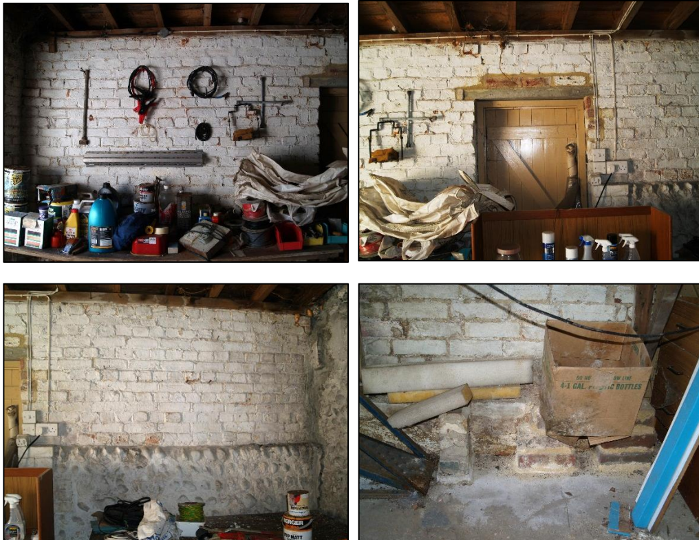
Plate 8 – The southern internal elevation of G1 shown from east to west (top left to bottom left) note the English bond brickwork and low flint wall at the western end (bottom left). Also detail of the earlier brick plinth at the base of the wall to the east of the door.
