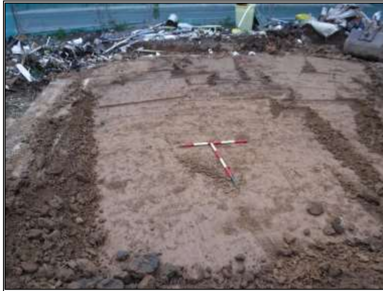
Plate 1: The Site after ground reduction, looking west
