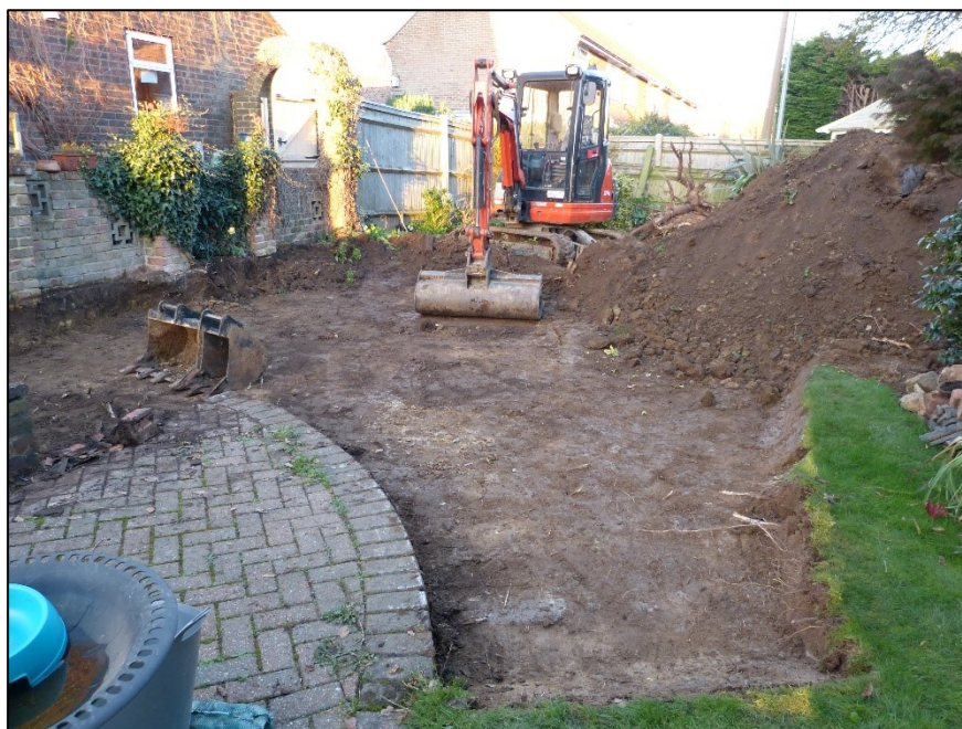
Plate 1: View across site during topsoil strip
