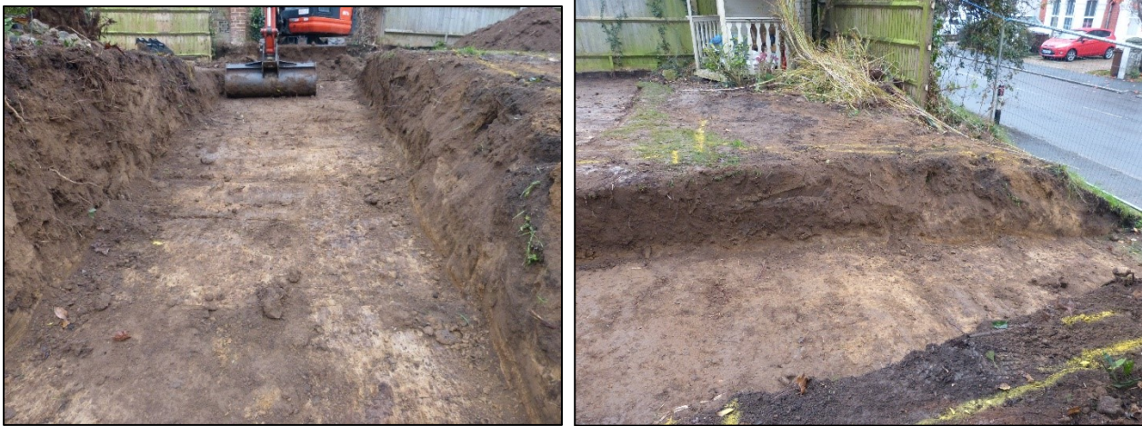
Plates 2 & 3: Access slope reduction revealing natural clay deposit
