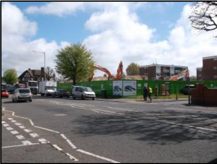
Plate 1:- View of site from Seaside.
