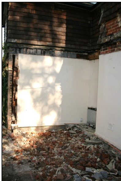
Plate 6: Wall Construction of Original South-Western Extension
