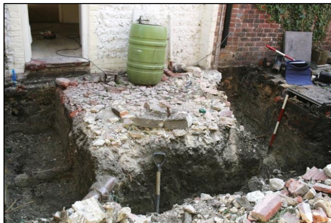
Plate 3: Completed Footings Trenches for Western Extension taken from the West
