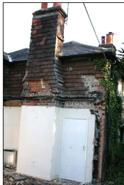
Plate 7: Original South Wall and Chimney Stack of Cottage
