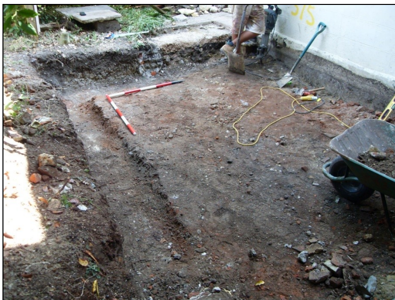
Plate 1: East facing shot showing excavated area and footing for the concrete raft.
