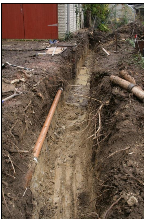
Plate 1: Excavated foundation trench for boundary wall
