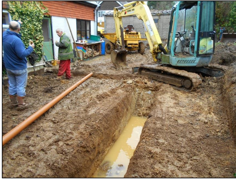
Plate 2: Excavated foundation trenches for extension
