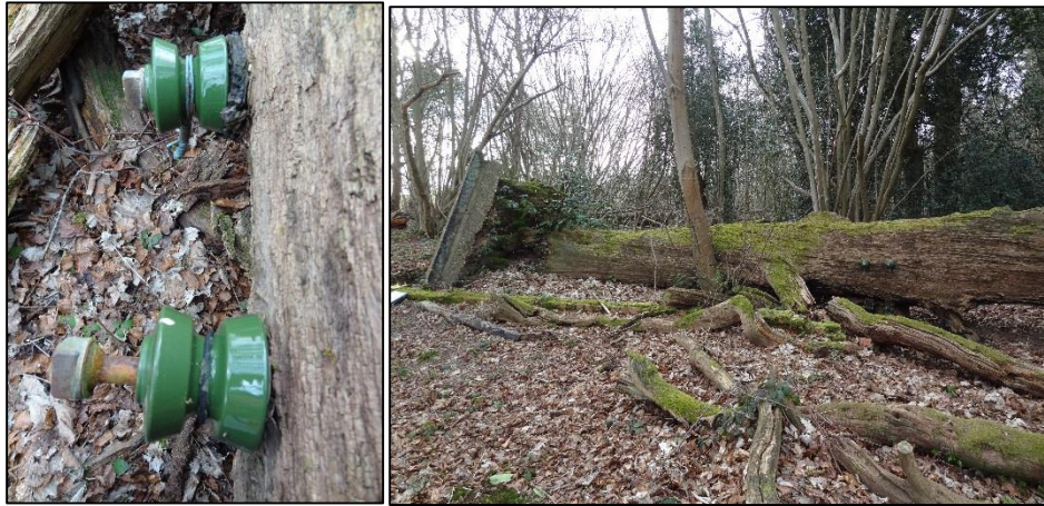
Detail of Ceramic Insulators on the fallen tree (above left), the fallen tree and uprooted concrete slab (above right).
