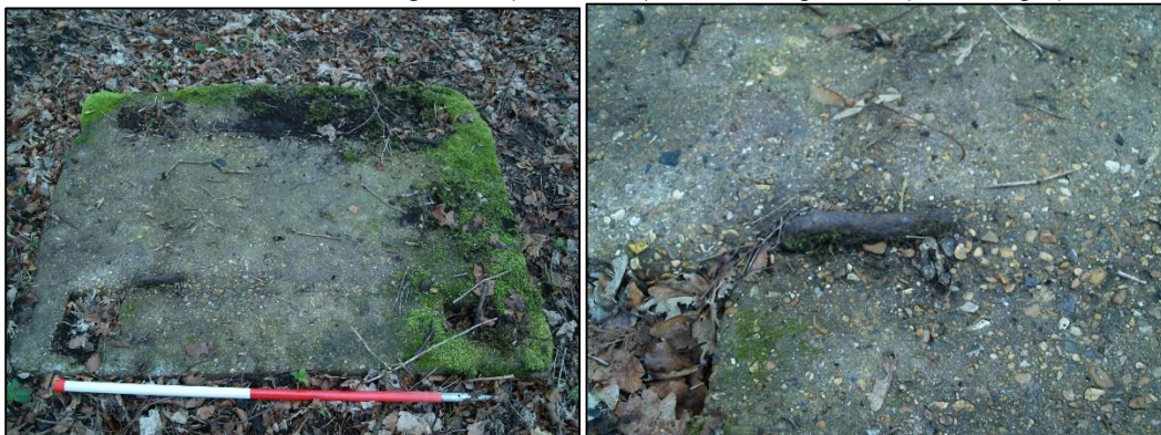
Concrete base to adjacent to the south end of SP.045 (above left) and detail of studs. (above right)
