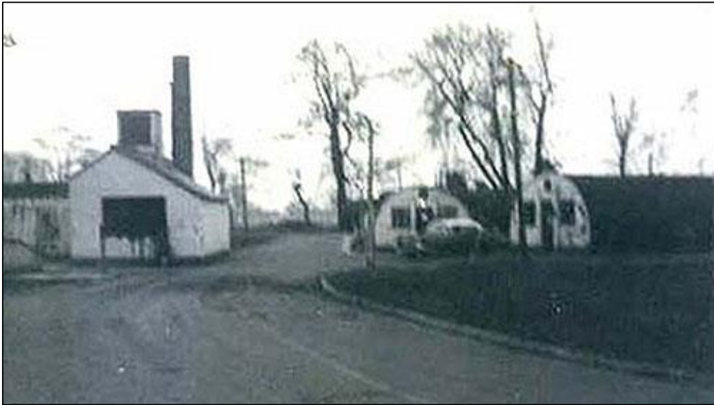
Plate 16 - An example of a Latrine/shower building associated with Nissen Huts
