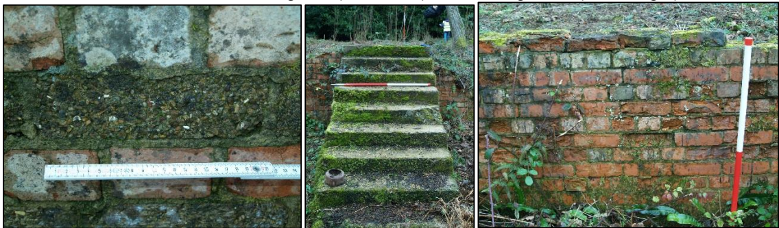
Detail of concrete 'brick' inclusions (above left), steps in south wall entrance with original kettle (above middle) and SW Wall showing variation in brick type (above right).
