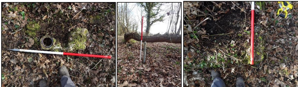
Plate 39 – Feature SP.063 showing the glazed drain (above left) the standpipe (above centre) and the concrete slab (above right).
