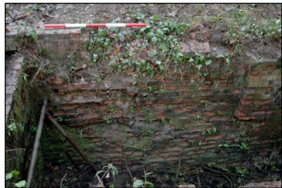
Plate 4: Eroded Brickwork South End of Western Wall (Context 1)
