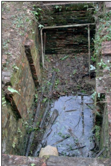
Plate 3: Brick Piers and Eroded Brickwork South Wall (Context 1)
