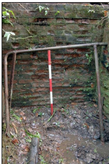
Plate 3: Brick Piers and Eroded Brickwork South Wall (Context 1)
