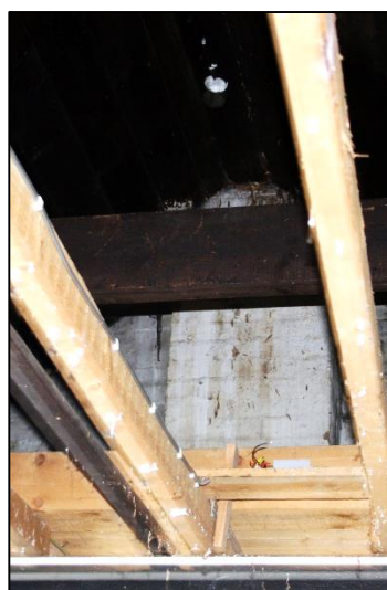
Plate 11: Brick Built Chimney Visible in Roof Space above G1
