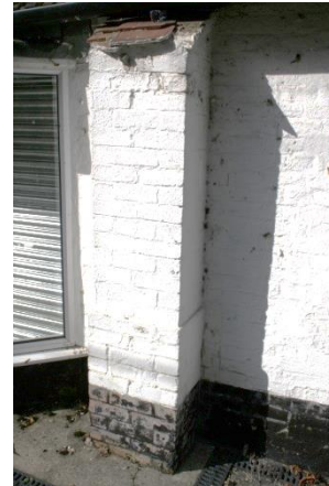
Plate 4: Sealed Chimney Stack
