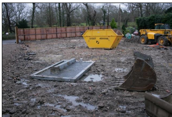
Plate 1: Site after Demolition of Buildings
