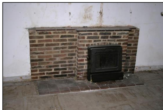
Plate 17: Modern Brick Built Fireplace G6
