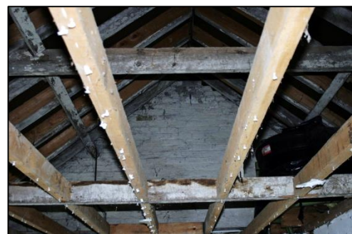
Plate 22: Roof Structure South End of main body of the Building
