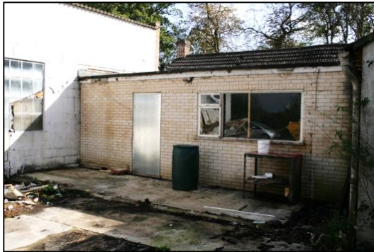
Plate 6: Northern End of Western Elevation taken from the South-West
