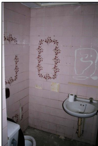
Plate 14: WC taken from Doorway in the Western Wall
