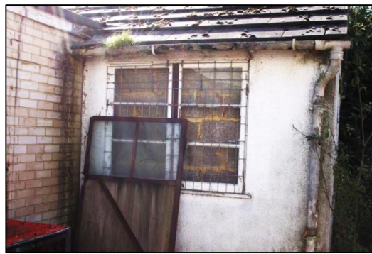
Plate 8: Window Sealed by Inserted Wall
