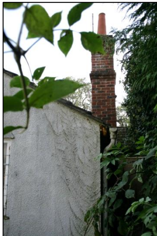
Plate 5: Chimney Stack Southern Elevation
