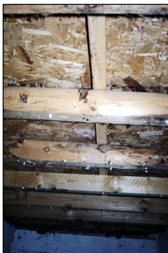
Plate 15: Ceiling of G4
