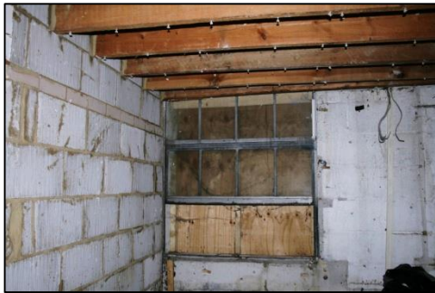
Plate 18: Garage Workshop Window in G7
