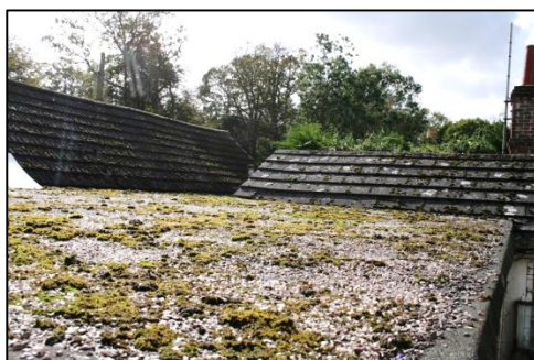
Plate 24: Flat Roof over Connecting Range
