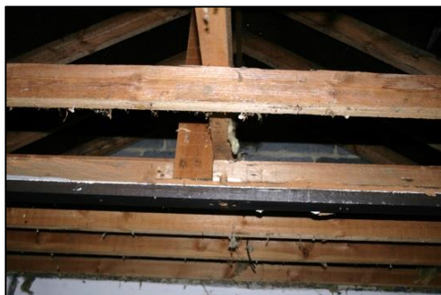
Plate 23: Roof Structure of the Originally Detached part of Building G6
