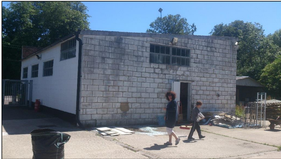
Plate 26: Garage taken from the west end
