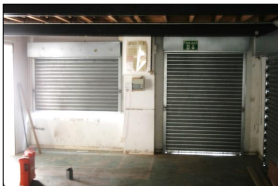
Plate 10: North Wall from Interior G1
