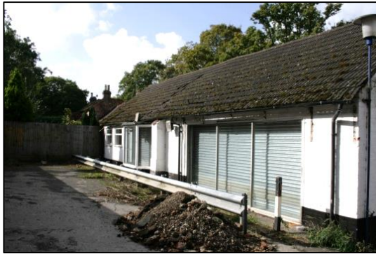
Plate 3: Western Elevation taken from the North-East
