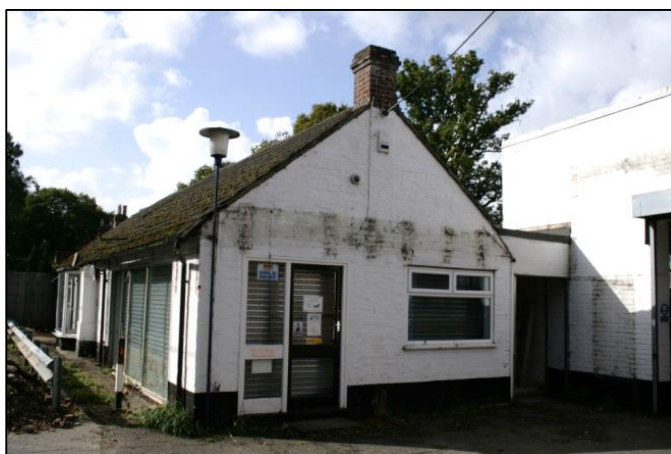
Plate 2: Northern Elevation taken from the North-East
