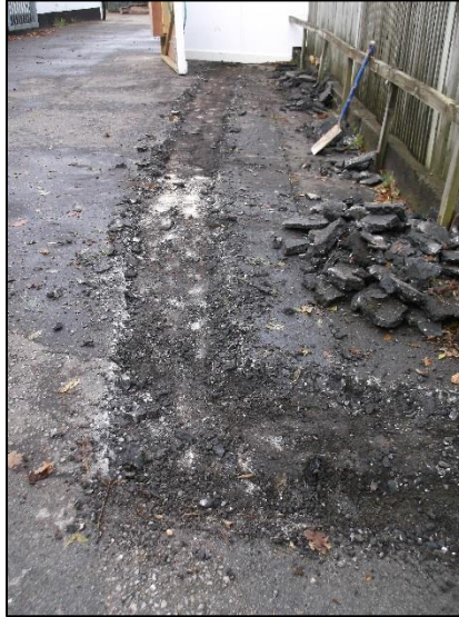
Plate 28: Abandoned service trench
