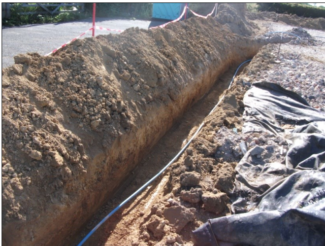
Plate 2: Trench 1, looking east
