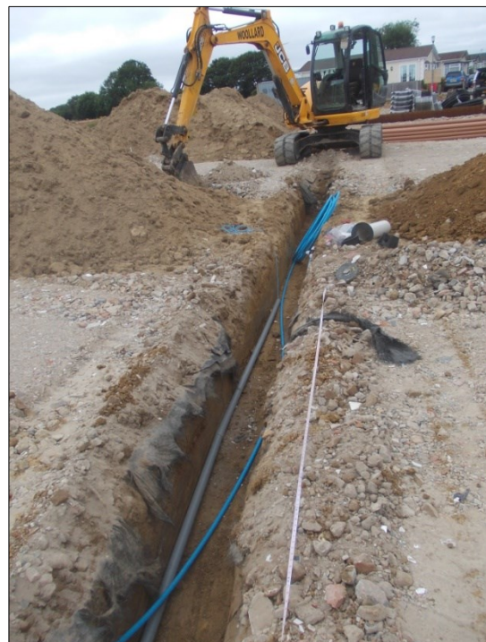
Plate 3: Trench 2, looking northwest
