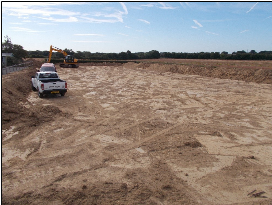
Plate 1: View across site after topsoil strip
