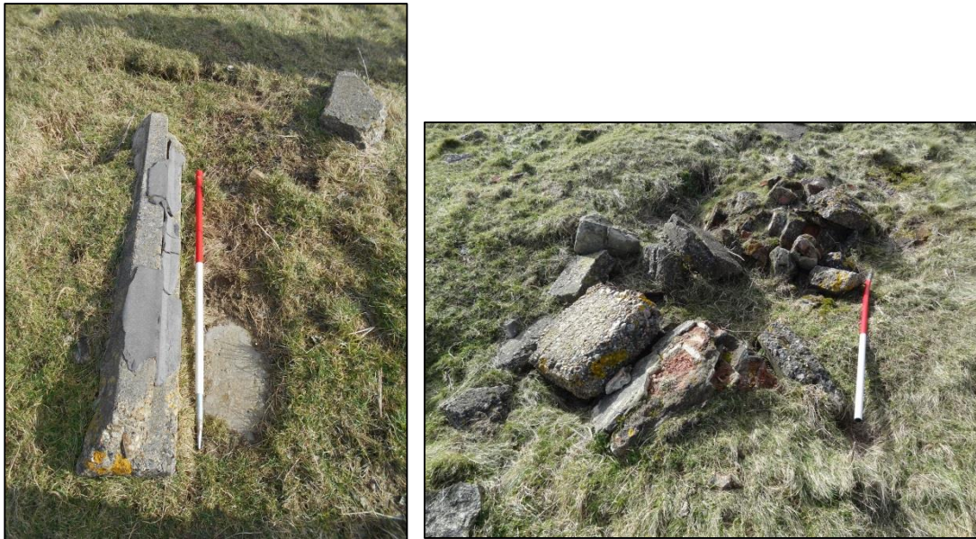
Plate 22: Concrete and other building debris relating to WW2 activity (GAY103 & 068)
