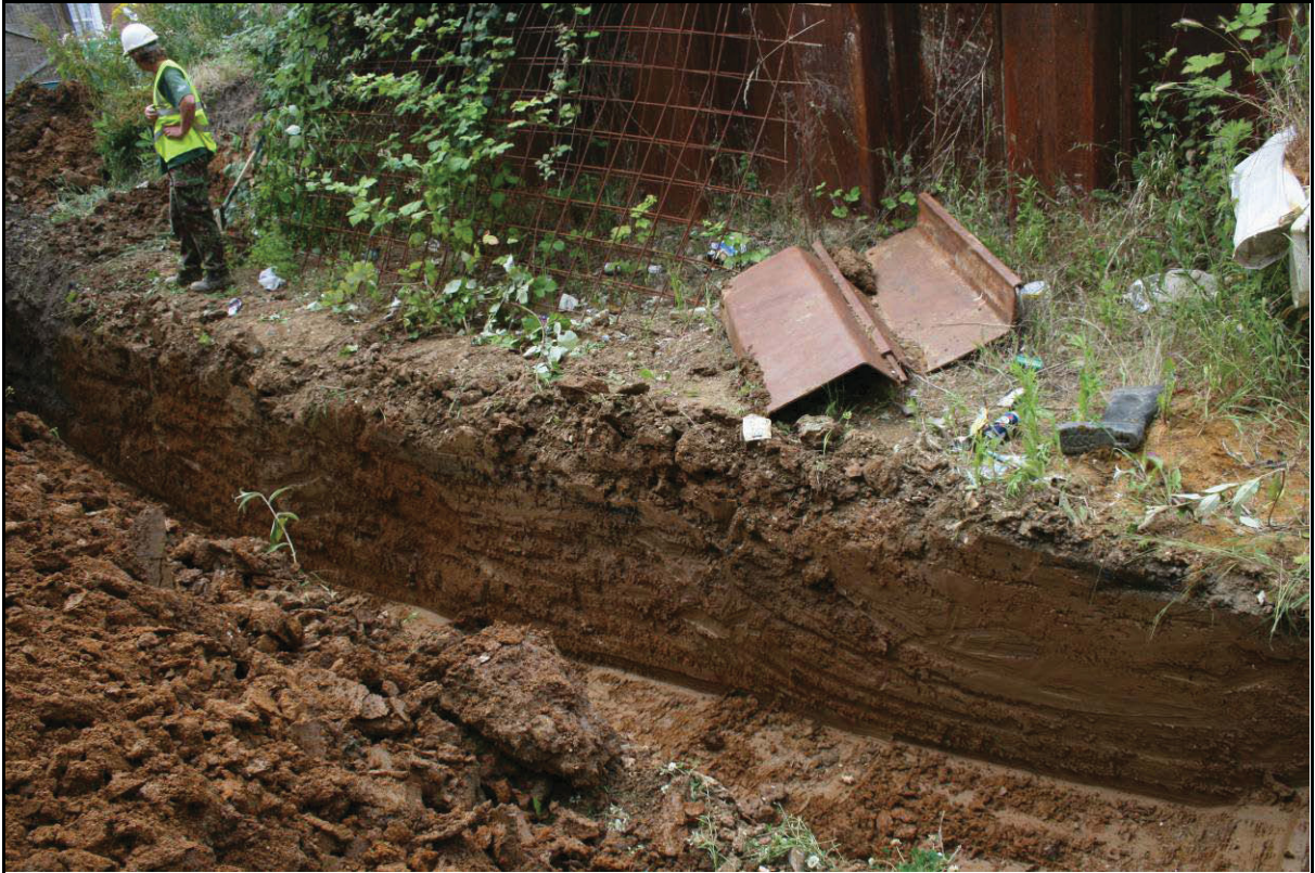
Fig. 7: 561A High Road, Ilford: Evaluation trench
