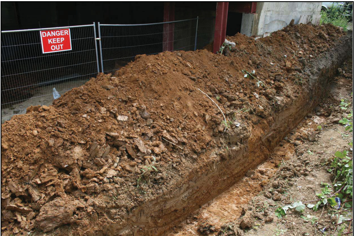
Fig. 8: 561A High Road, Ilford: Evaluation trench
