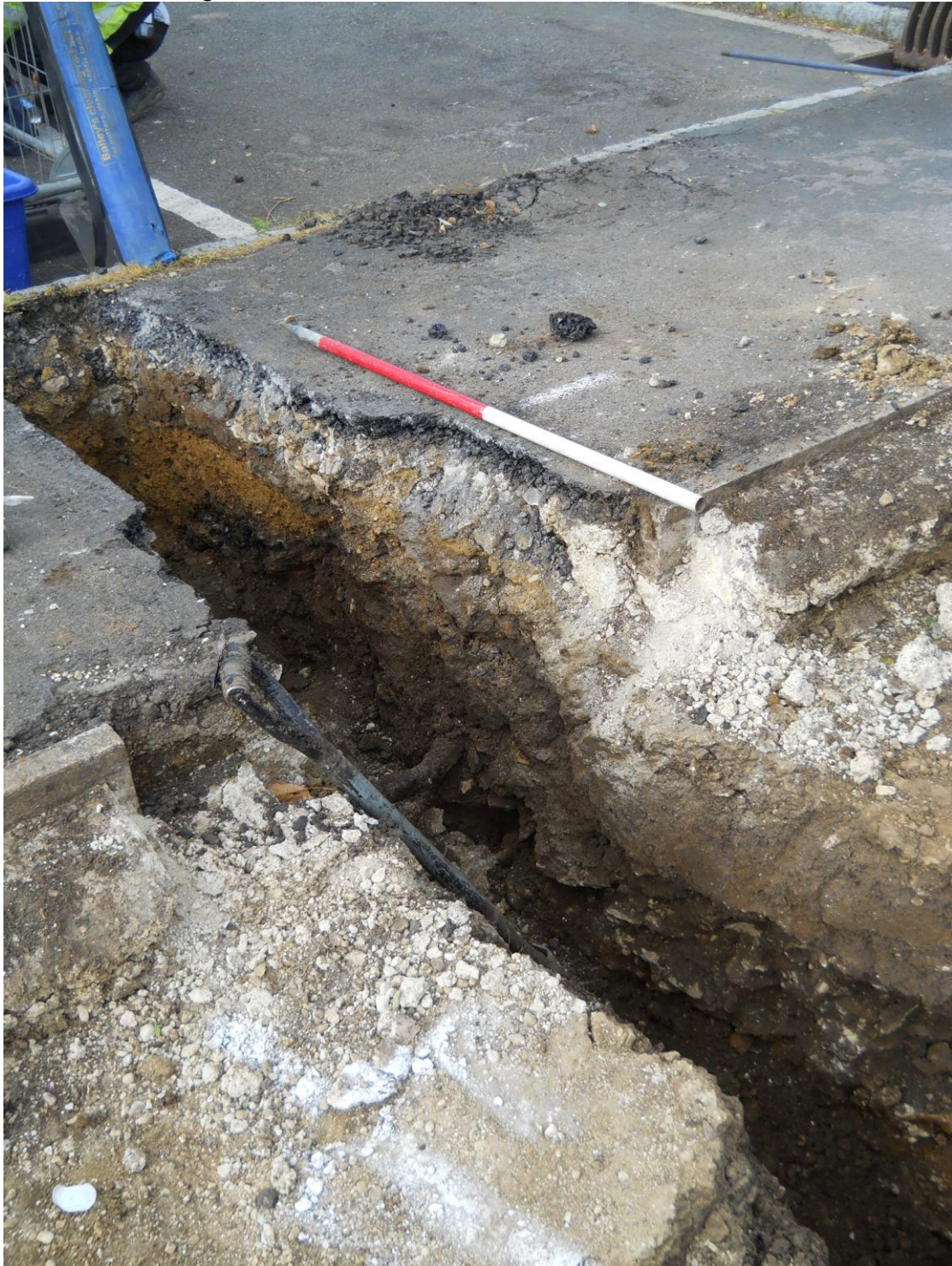
Plate 1: South facing section of trench excavation
