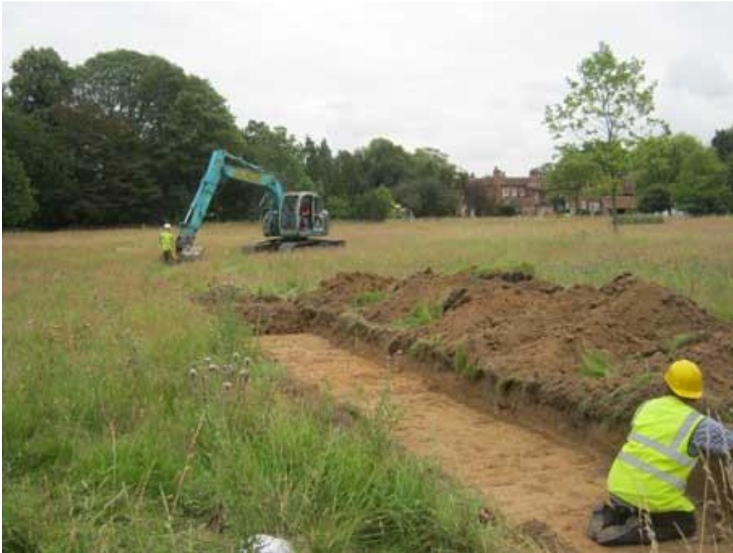
Figure 3. General view of the Site looking south towards Paradise House showing machining, and section recording of Trench 5 in progress.
