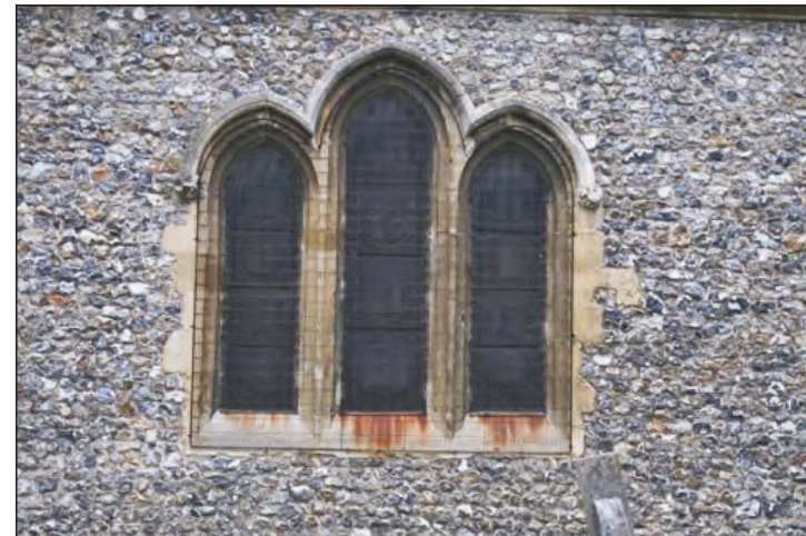
Plate 6. Phase 3, surviving triple lancet window in south aisle
