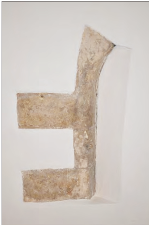
Plate 7. Phase 3, remains of partial doorway in south aisle
