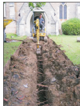
Plate 5. Drainage Trench looking north
