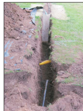
Plate 6. Drainage trench looking south west
