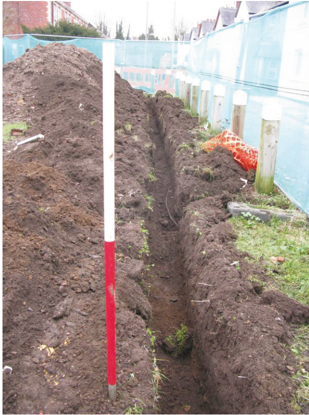
Plate 1: General shot of Electricity cable trench
