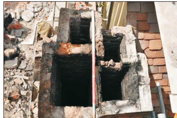
Plate 9. Middle section through chimney
