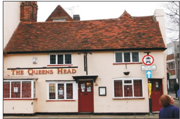
Plate 2. General view of Queen's Head front facade
