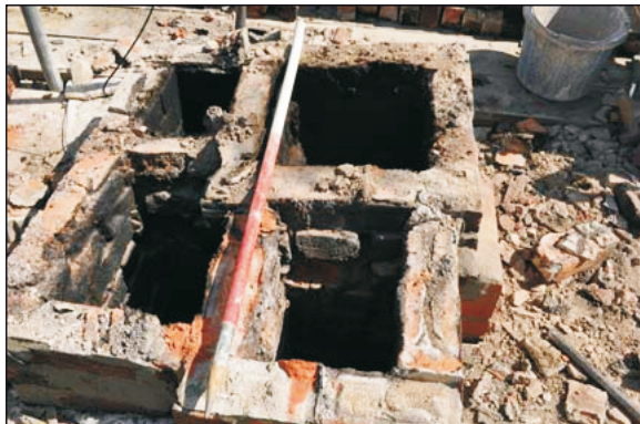
Plate 8. Upper section through chimney
