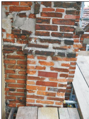
Plate 5. Detail on chimney
