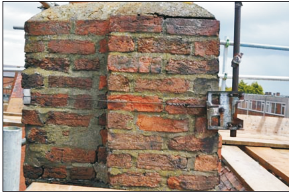
Plate 6. Detail on chimney
