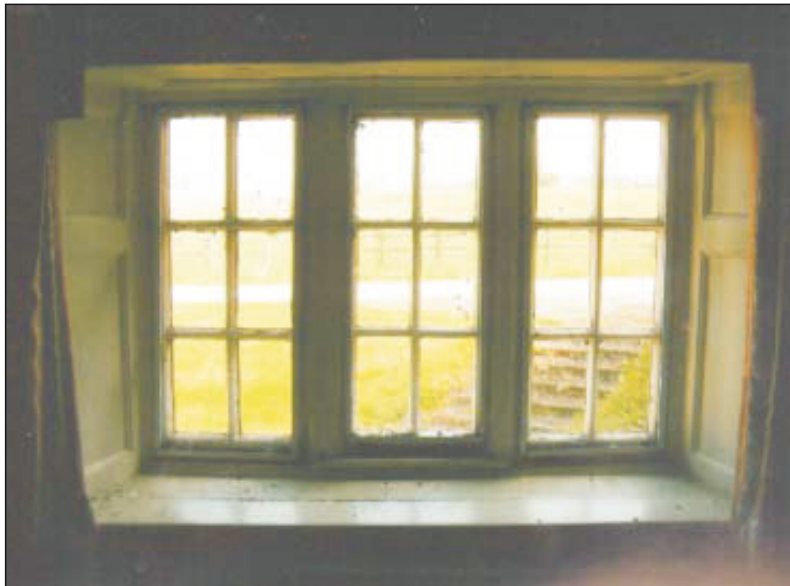
Plate 22: First phase two light window (to the right) mullioned window in rear (north elevation) at first floor.
