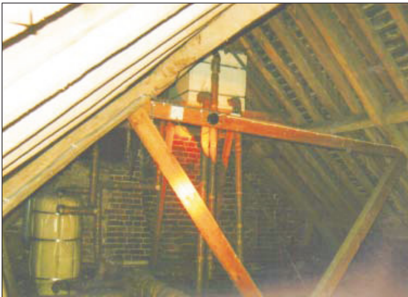
Plate 28: Roof over phase 2, looking east.
