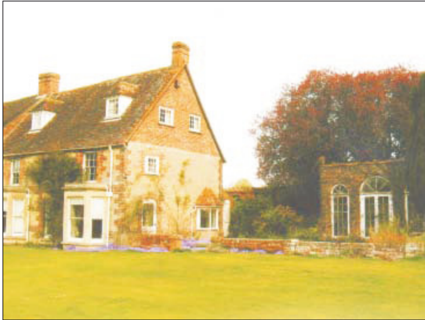
Plate 3: House from the south east. Note the brick gable which may have formerly been hipped.
