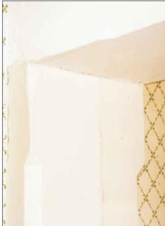
Plate 25: First floor, east room. 18th century (?) boxed beams.
