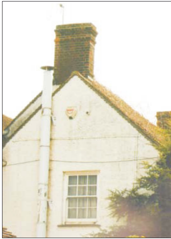
Plate 15: West gable of late extension.
