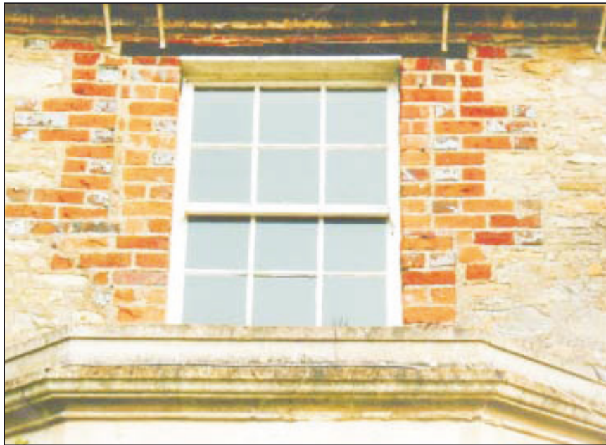
Plate 7: First floor window in south front. West end of first phase.
