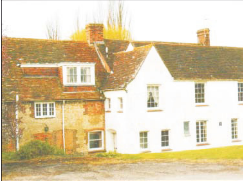
Plate 13: North elevation showing first phase house to left (east) and gabled second phase stair turret centre.
