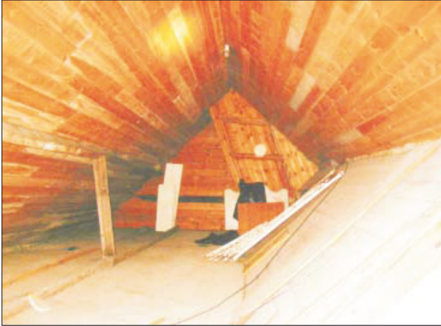
Plate 31: Further western extension roof, showing sarking boards, looking east.
