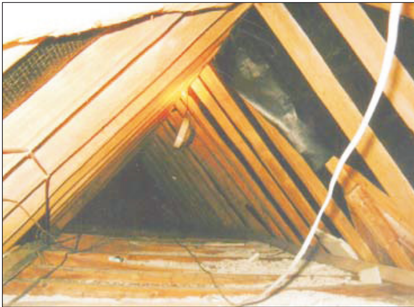
Plate 27: East roof looking east.
