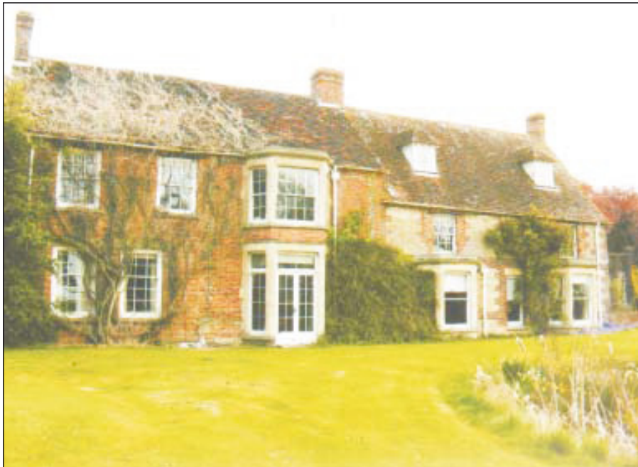
Plate 1: South front. Note 17th century wing to right, also one bay of 18th century work to left and 19th century extension to left of this.
