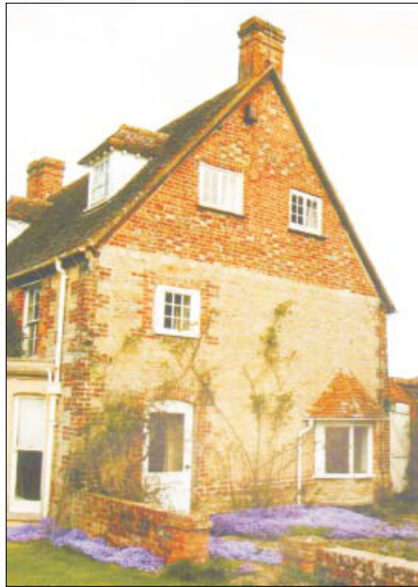
Plate 5: East gable. Note the brick quoins and rounded jambs of doorway.
