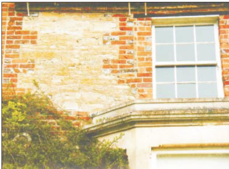
Plate 8: First floor window in south front. Note that the window was formerly wider and shorter.
