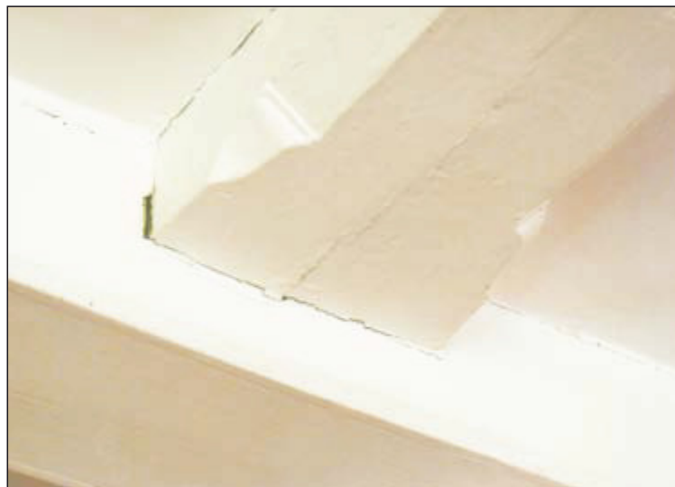
Plate 20: Stopped and chamfered summer beam in south east first floor.
