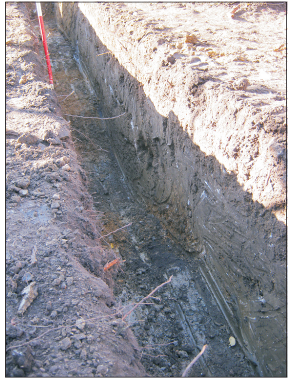
Figure 4. Photograph of footings trench looking northwest
