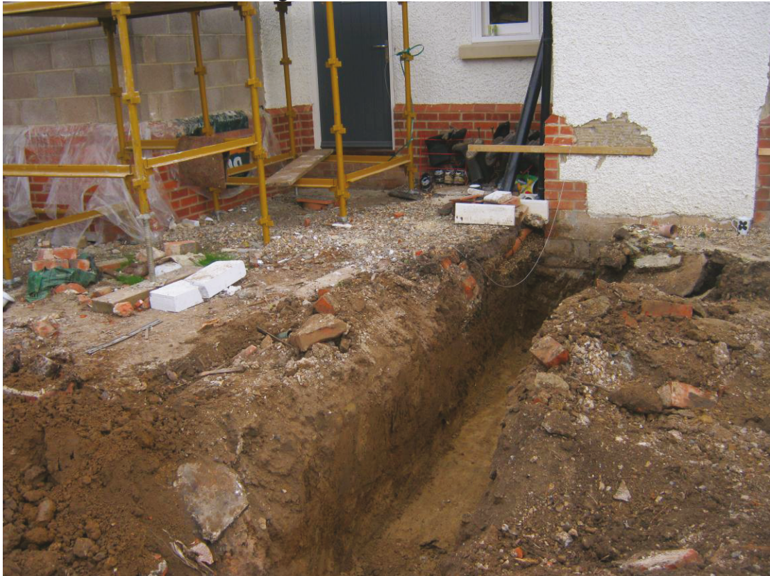
Plate 2: General view of footing trench; rear extension
