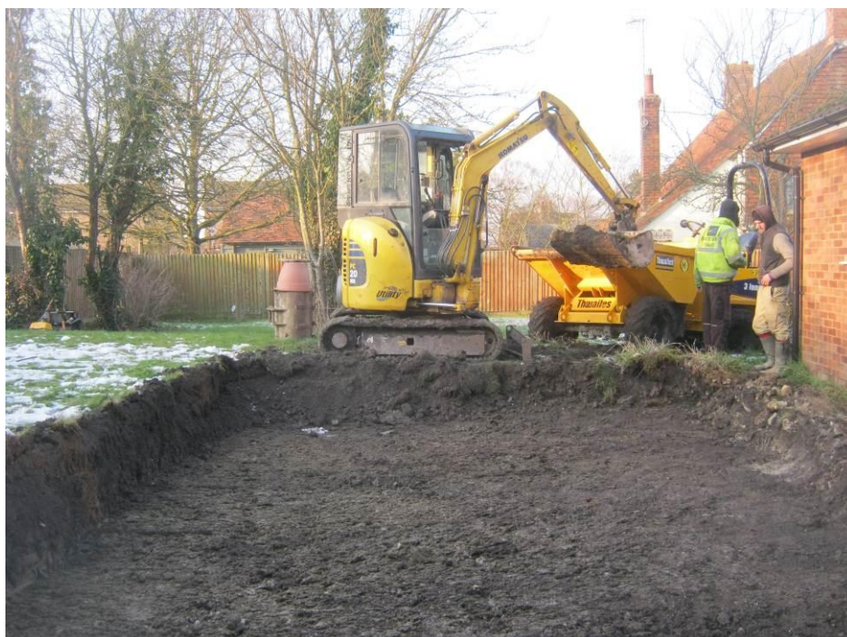
Figure 2. Machine excavation of the western area of the Site.
