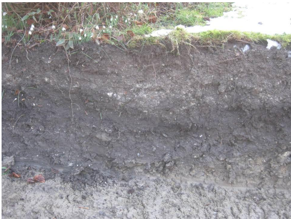
Figure 3. East-facing section of the western area of Site, with redeposited mixed material above the original topsoil. The natural subsoil is visible at the bottom of the section.
