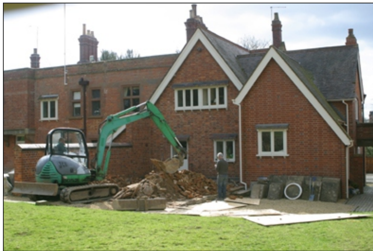
Figure 10. North wing, looking southeast (2012).
