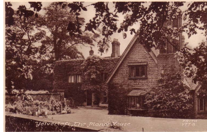
Figure 11. North wing, looking southeast (1955).
