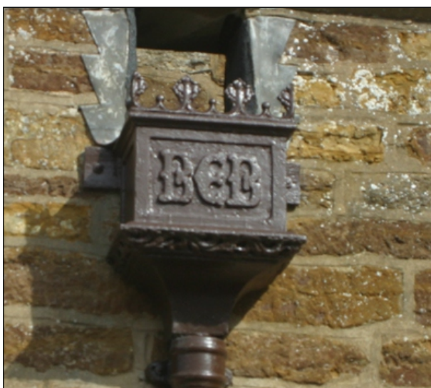
Figure 5. Cast-iron down-pipe with BEB initials.
