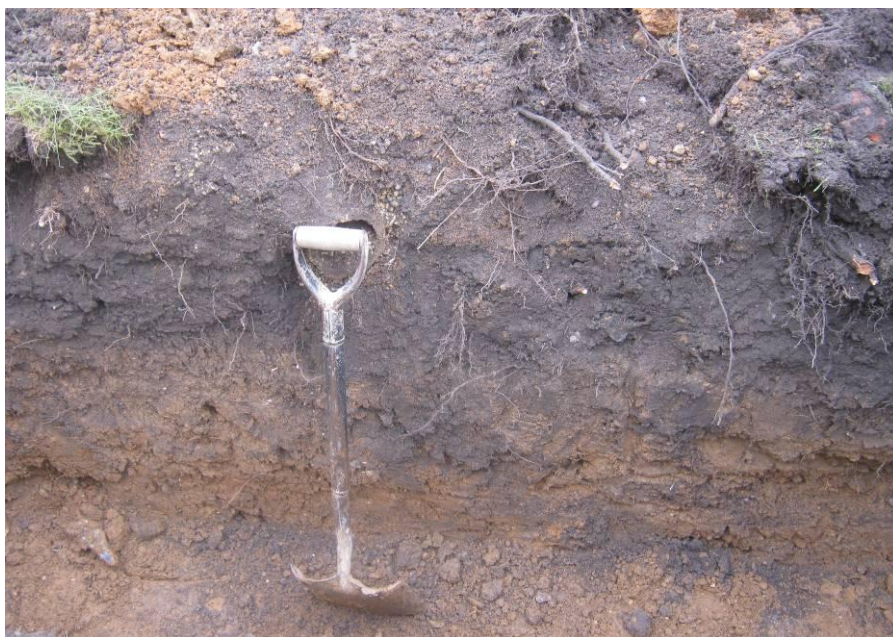
Figure 3. Representative section of the footings trench.
