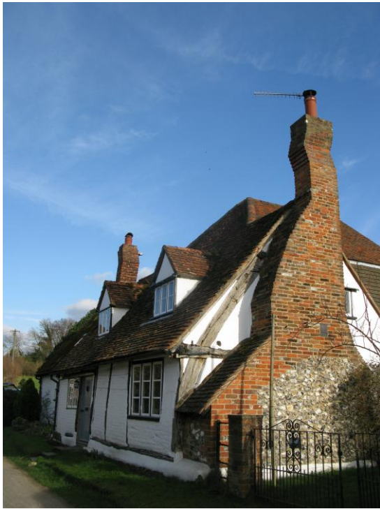
Figure 3; Crooked Chimney Cottage
