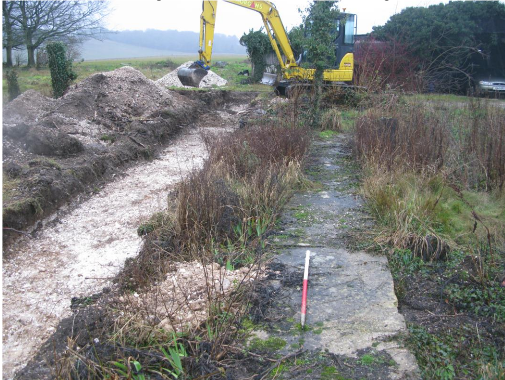
Plate 3; Concrete kerbing assumed to be associated with the previous windmill
