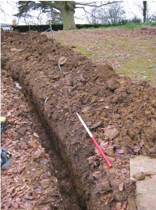
Figure 3: General view of Electricity Cable Trench looking west
