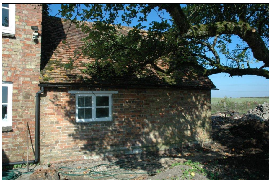
Fig 2. The east elevation of the two extensions, showing the block bonding of the two.
