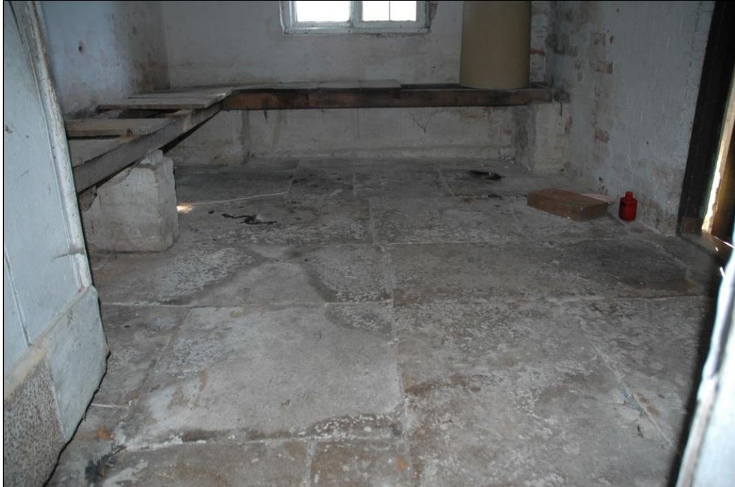
Fig 4. The 'Cold Store' flagstone floor and wooden benches on brick piers. Also showing is the door on the left hand side, repaired at its foot.
