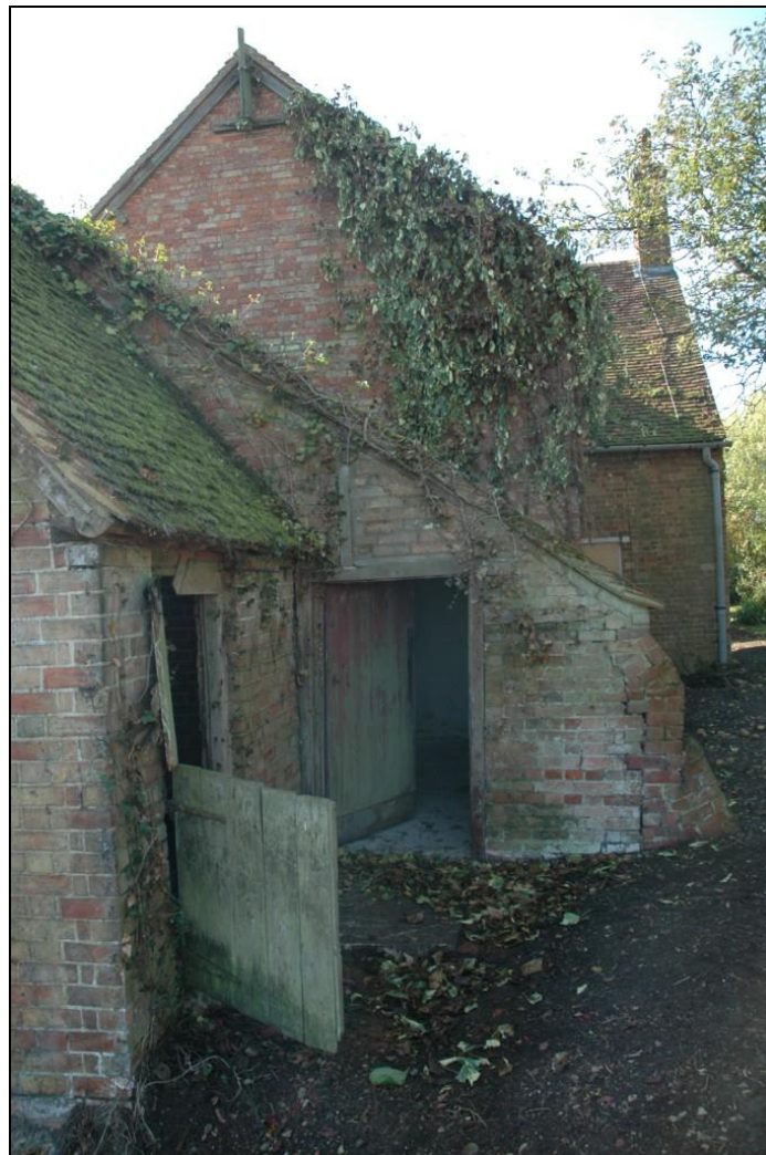
Fig 3. View from the north-west, showing the split-leaf door to the stable (left) and inserted hayloft and the door to the larder (centre) leading on through to the 'Cold Store'.
