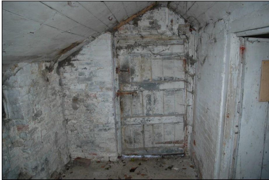
Fig 6. The lean-to representing the second phase of construction.
