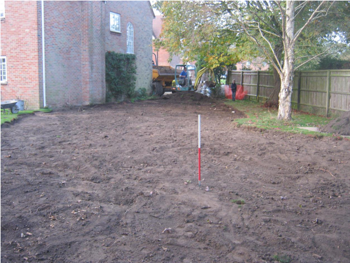
Plate 1: General; Topsoil strip looking north.
