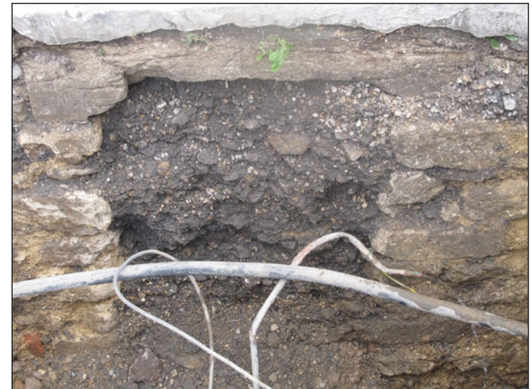
Figure 6. Photograph above showing close-up of access in wall 105.
