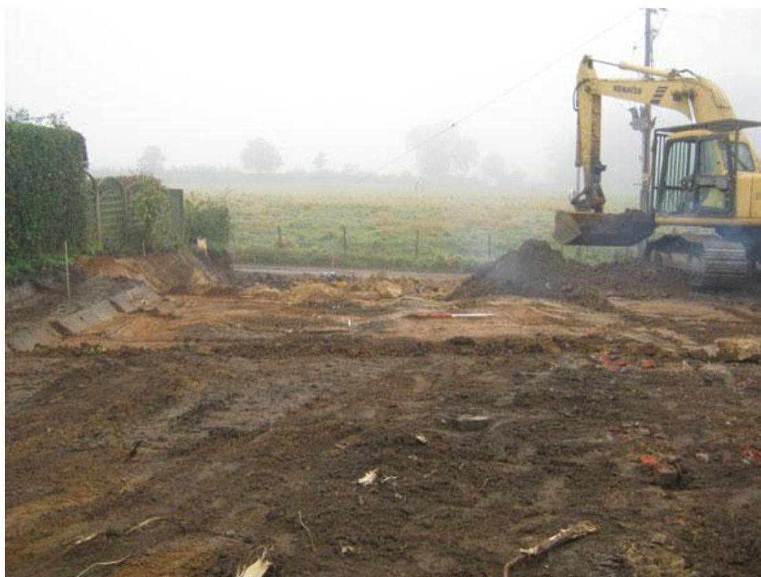
Figure 2. Ground reduction over area of new build
