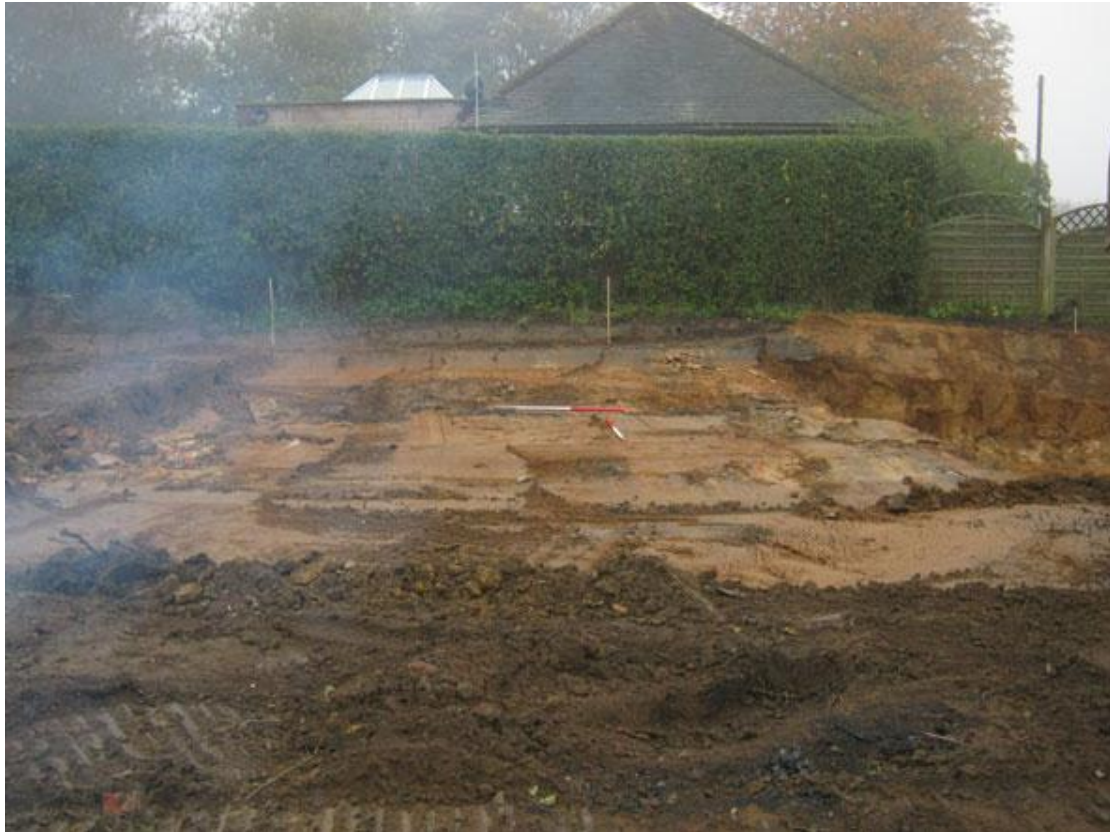
Figure 3. Ground reduction beneath former house; excavation to right.
