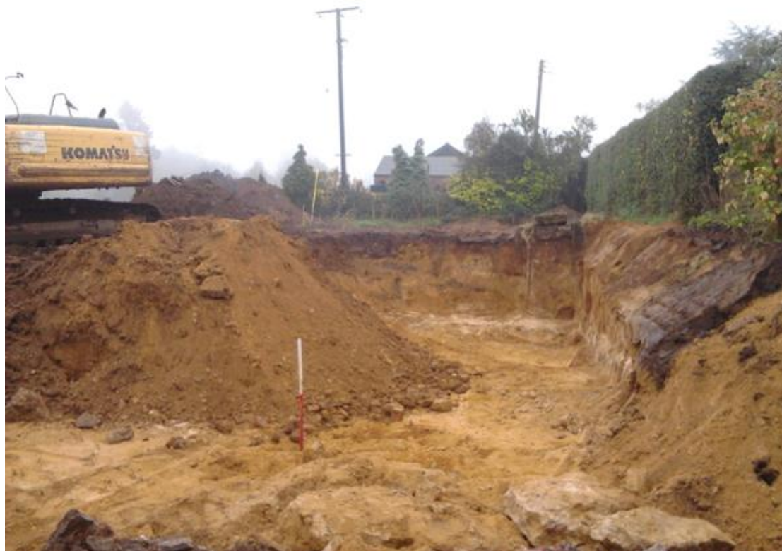
Figure 4. Investigation area following excavation
