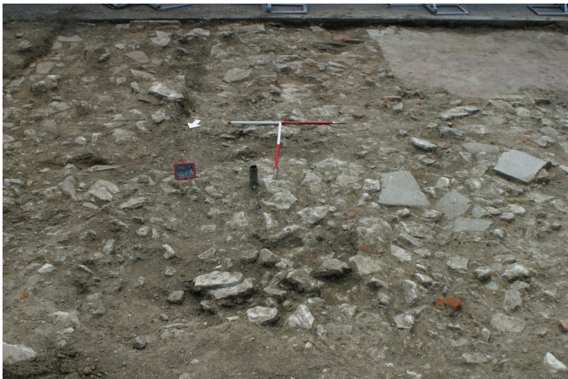
Figure 6; General view of Area A looking south (1m scales) showing demolition deposits
