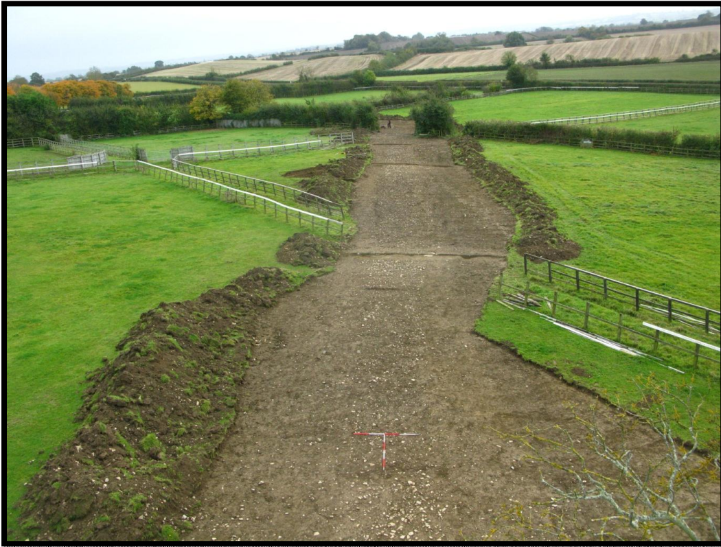
Plate 4; View of Road looking south-east (2m scales x2)
