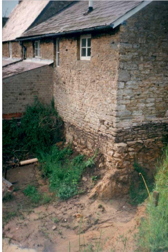
Plate 1; Showing corner of 1 Church Street previous ground reduction
