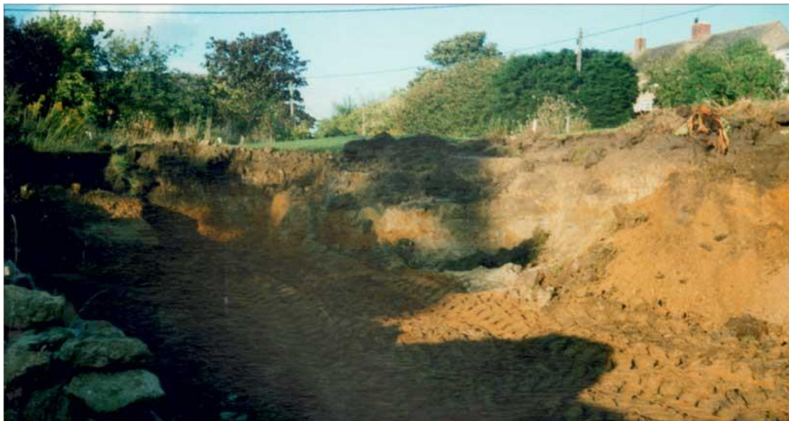
Plate 2; Showing extent of some of the previous groundworks in the garden
