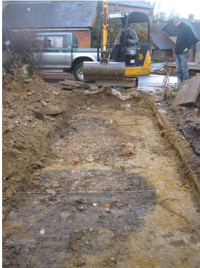
Figure 3. Machine excavating Trench 1, looking north-west, with pit cut 101 in the foreground.
