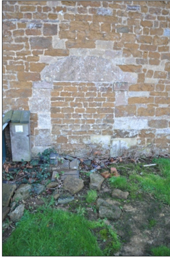
Plate 8. Blocked Norman, 12th century doorway
