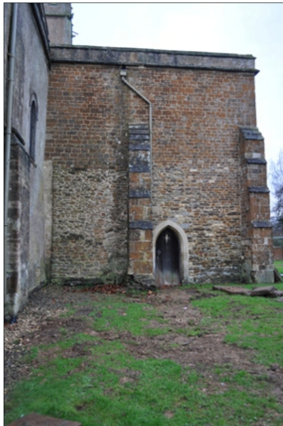
Plate 7. North wall of transept containing part of the Norman arch into the chapel
