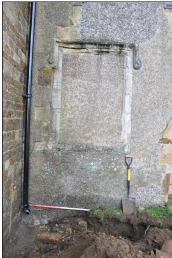
Plate 2. Wall 19 in context to the rest of the elevation
