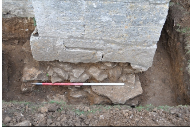
Plate 3. Wall 23 under buttress, from south
