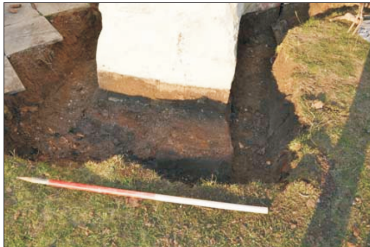
Plate 2. South west buttress on tower
