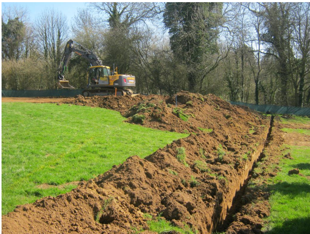
Figure 2. View of machining taking place on the Site with the service trench visible in the foreground, looking east. Note the significant break in slope.
