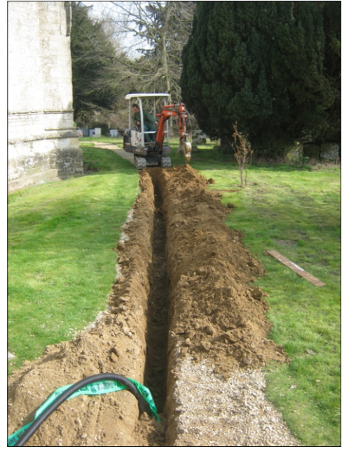
Plate 2. Machine excavation of trench, looking Southwest.
