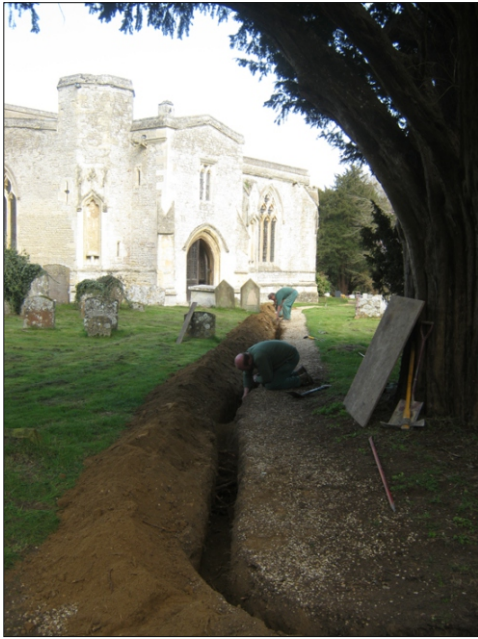
Plate 1. Hand excavation of trench, looking Southwest.
