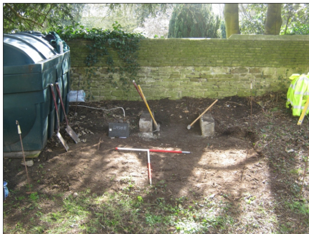
Plate 4. Excavated footing for concrete base, looking Northwest.
