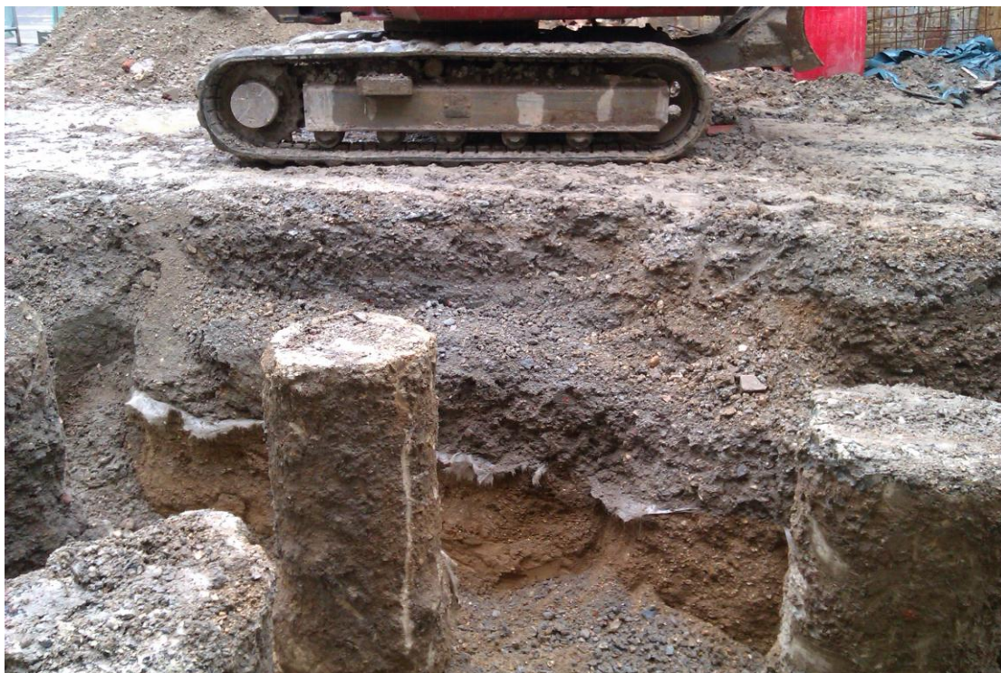
Figure 2. North end of ground reduction area round piles; looking south.
