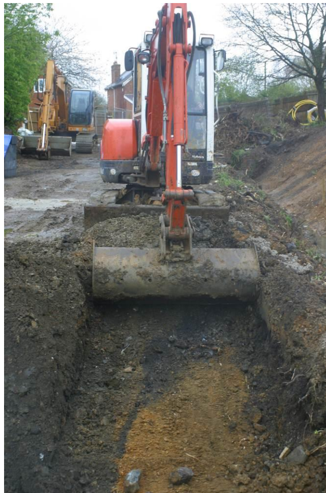
Figure 3. Machining on Site on the 18 th April 2012 looking north-east, in the western trench alongside the existing drainage ditch. The line of the modern electricity cable cut is visible at the left side of the trench, and the earlier drainage cut at the right.
