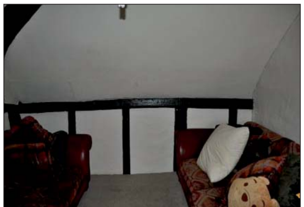
Plate 6. Internal timber frame upstairs rear
