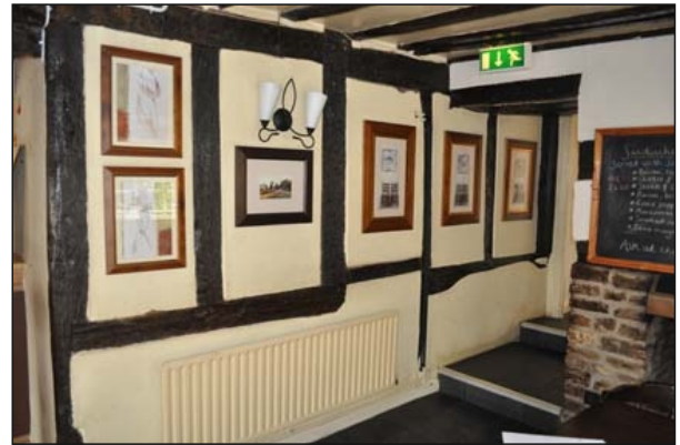
Plate 10. Internal timber frame downstairs rear
