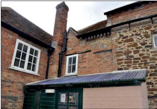
Plate 3. Dormer Window on North facade
