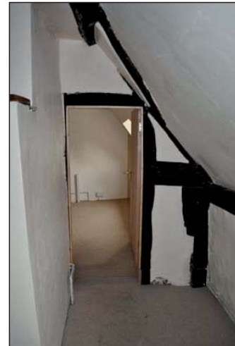
Plate 4. Internal timber frame upstairs rear
