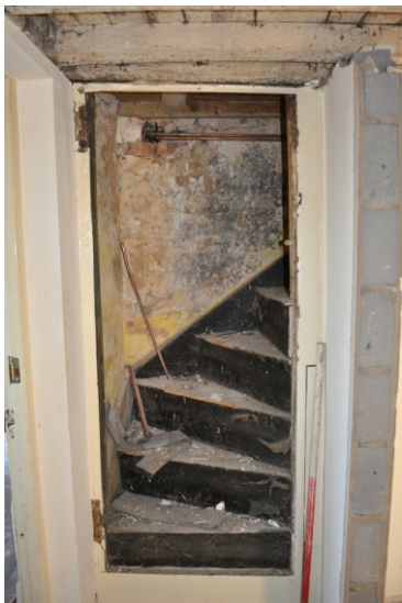
Plate 20. Spiral staircase, Structure A
