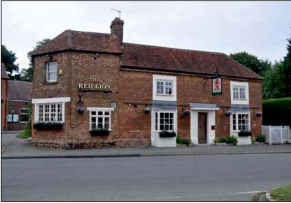
Plate 1. South and West facade of Red Lion
