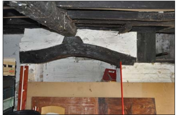
Plate 16. Fireplace lintel and axial beam Structure B
