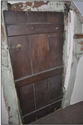
Plate 7. Internal timber frame upstairs rear
