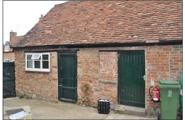
Plate 14. Structure B South facade
