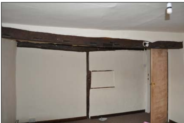
Plate 11. Beams and timber frame upstairs front
