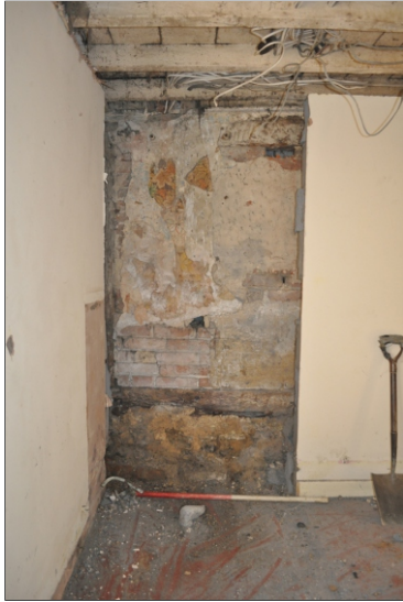
Plate 18. Timber frame wall forming part of Cruck, Structure A
