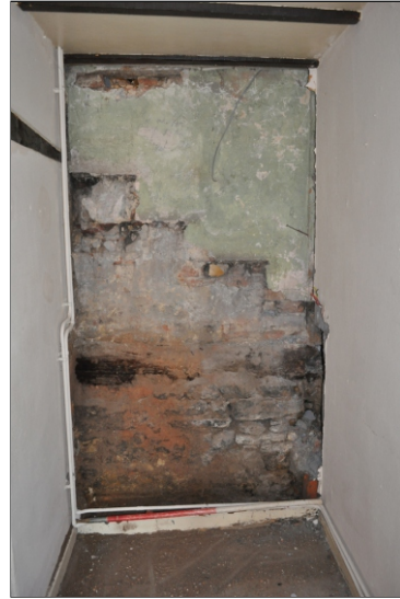
Plate 19. Timber frame wall forming part of Cruck, Structure A
