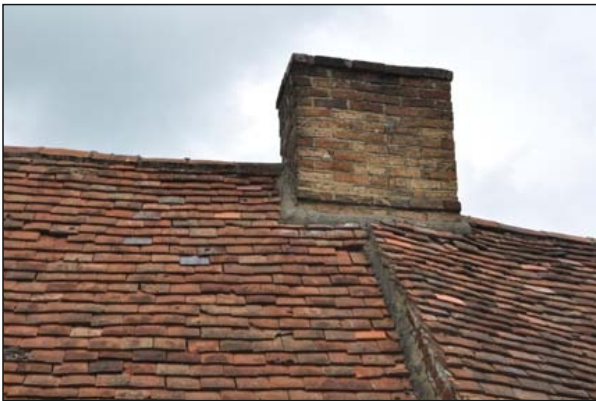
Plate 15. Chimneystack Structure B
