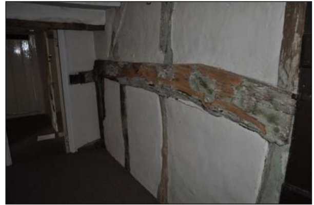
Plate 8. Internal timber frame upstairs rear
