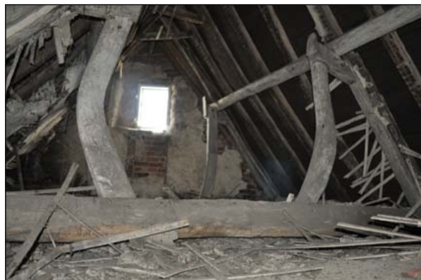
Plate 17. Structure B roof trusses
