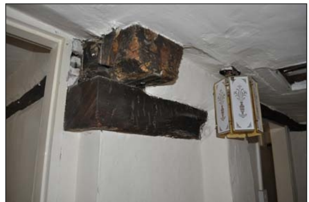
Plate 12. Plate and transverse tie beam
