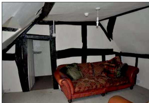
Plate 5. Internal timber frame upstairs rear
