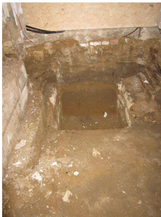
Figure 2. Underpinning pit showing stratigraphic sequence
