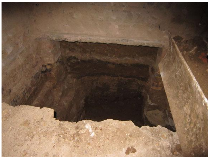
Figure 3. Underpinning pit showing wall construction technique
