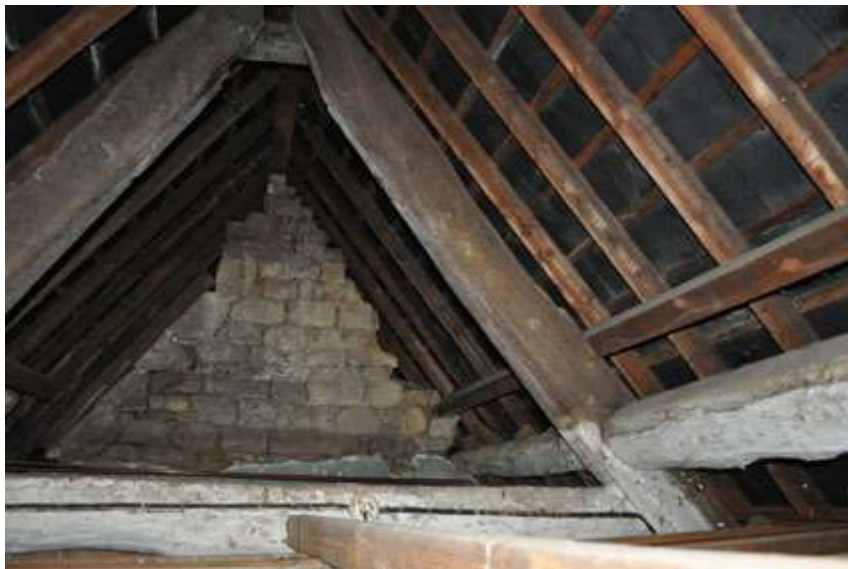
Plate 8 A-frame and chimney remains in attic over back bar
